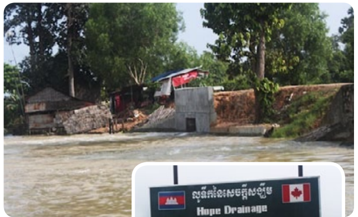
Above: This picture shows the extent of the flooding that the new Dam is keeping at bay.
